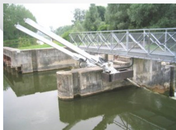
Mechanical jack on weir gate
