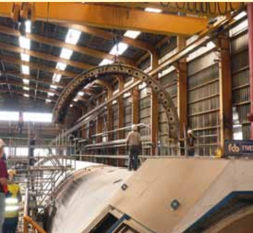
Riding tires used on sugar beet diffuser
